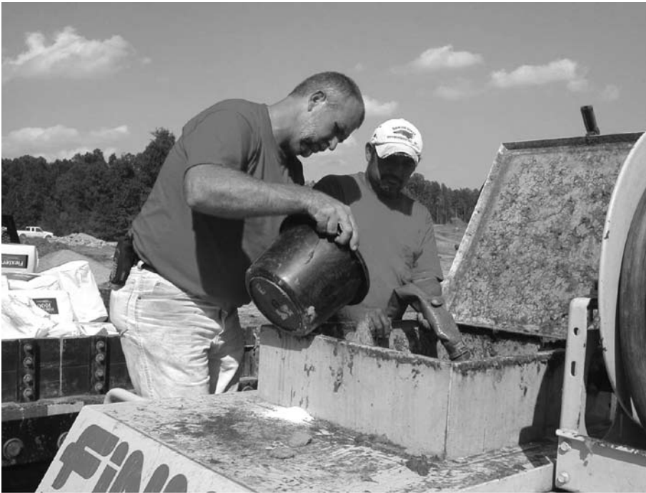
Figure 2. Granular PAM is slowly added to a hydroseeder tank under full agitation.
