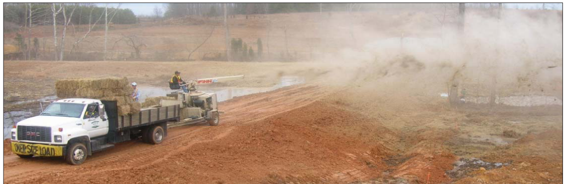
Figure 1. Applying straw with a blower pulled by a straw supply truck.
