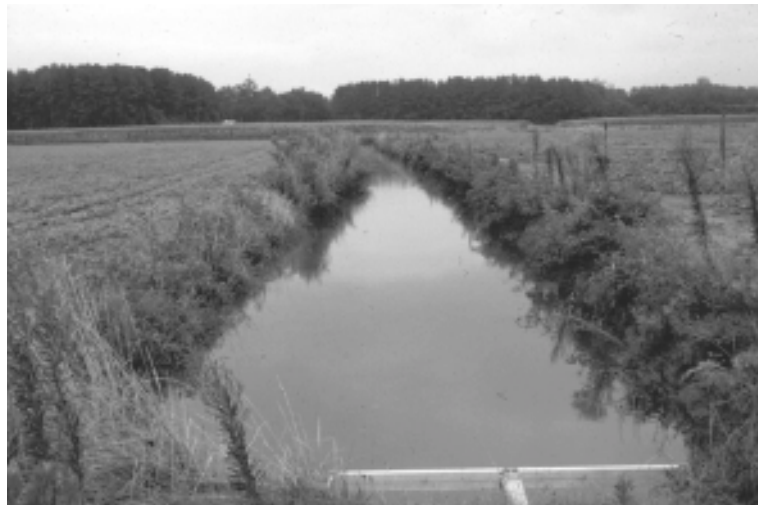
Figure 9b. Water profile in drainage ditch upstream of flashboard riser (see 9a).
