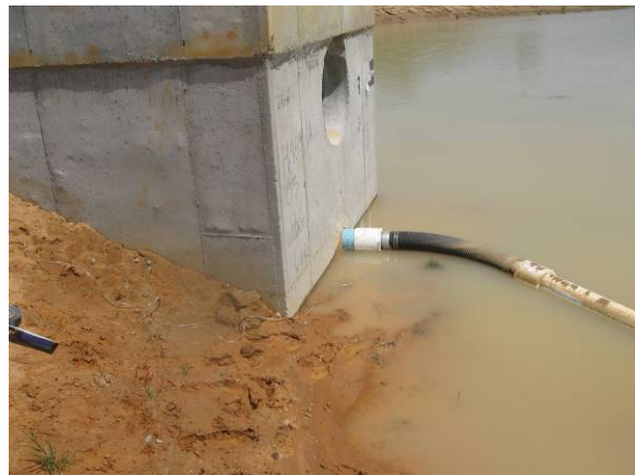
Figures 20 and 21. The large sediment basin and concrete riser outlet with skimmer.
