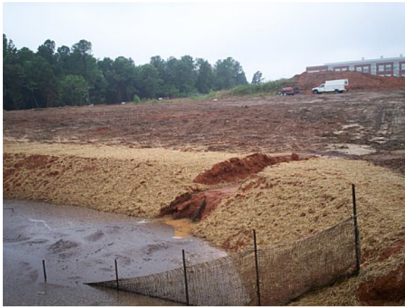
Figures 16 and 17. The disturbed area upslope and the sediment basin at Site WAKE2.
