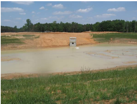
Figures 20 and 21. The large sediment basin and concrete riser outlet with skimmer.
