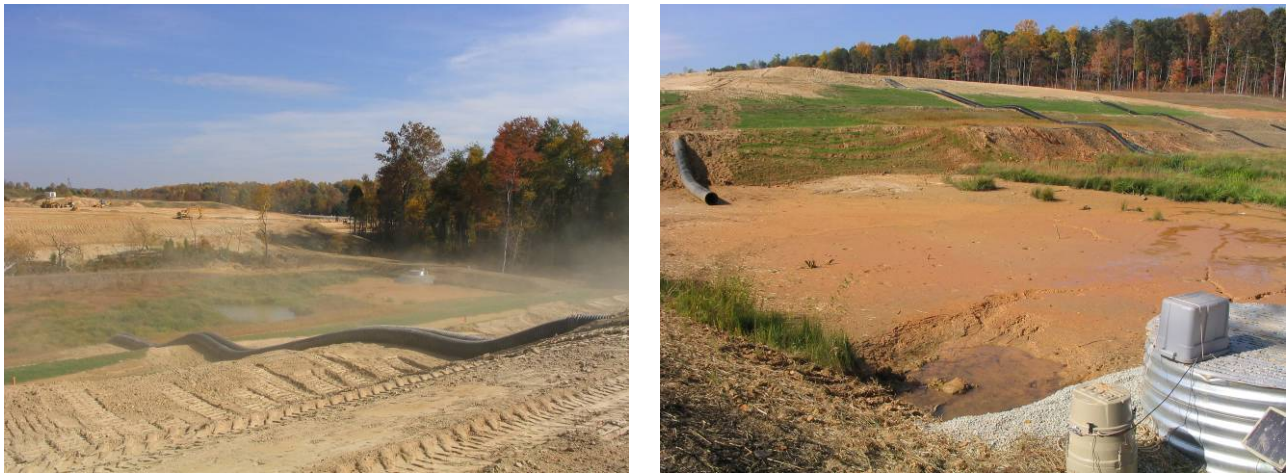
Figures 8 and 9. The disturbed area upslope and the sediment basin at Site GUIL.
