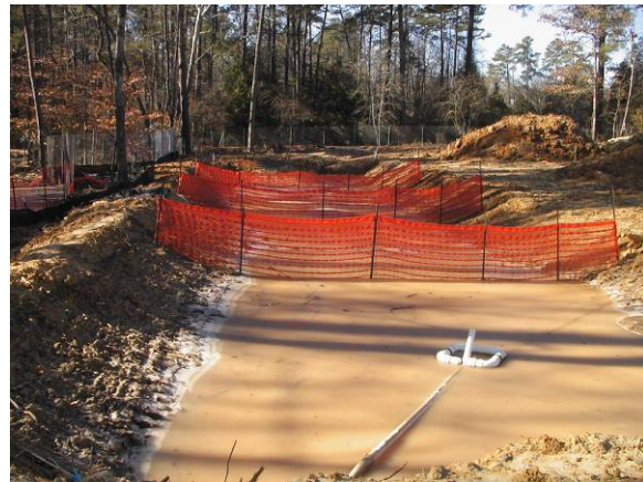
Figures 10 and 11. The disturbed area upslope and the sediment basin at Site ORAN.
