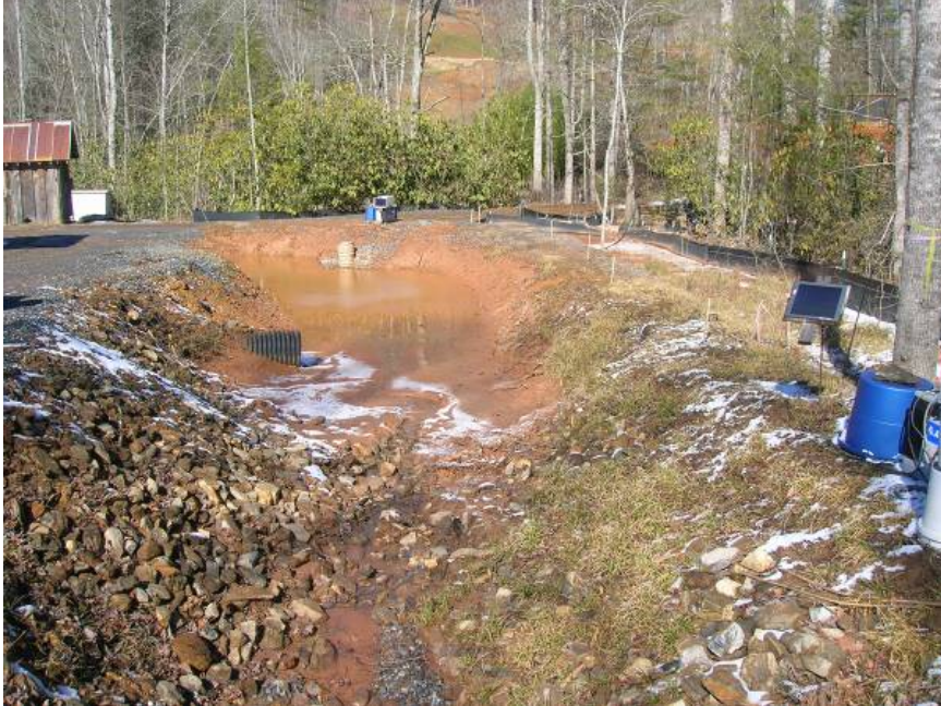
Figure 5. The sediment basin and samplers at Site JACK.
