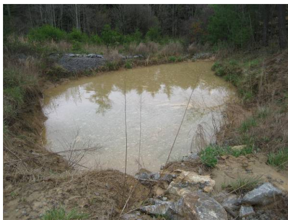
Figures 6 and 7. The disturbed area upslope and the sediment basin at Site BUNC.
