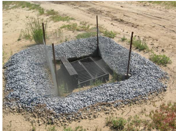
Figures 18 and 19. The disturbed area upslope and an example inlet structure at Site GREE.
