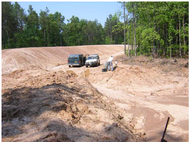
Figures 12 and 13. The upslope disturbed area and sediment basin at Site DURH. The photo on the right shows an attempt at maintenance, with a small amount of sediment removed and a new rock dam.
