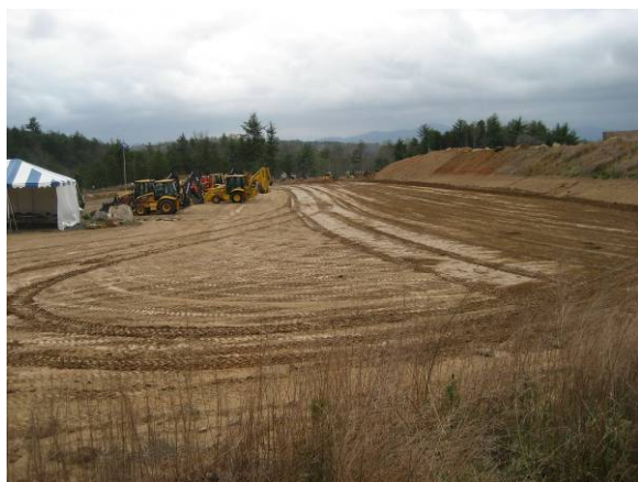
Figures 6 and 7. The disturbed area upslope and the sediment basin at Site BUNC.
