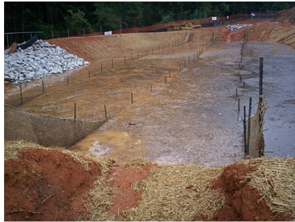
Figures 16 and 17. The disturbed area upslope and the sediment basin at Site WAKE2.
