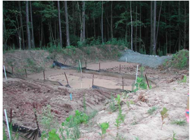
Figures 12 and 13. The upslope disturbed area and sediment basin at Site DURH. The photo on the right shows an attempt at maintenance, with a small amount of sediment removed and a new rock dam.
